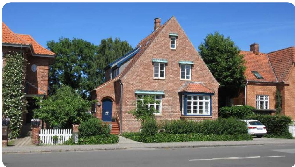
Carl Baggers Allé 27 i 2018.
